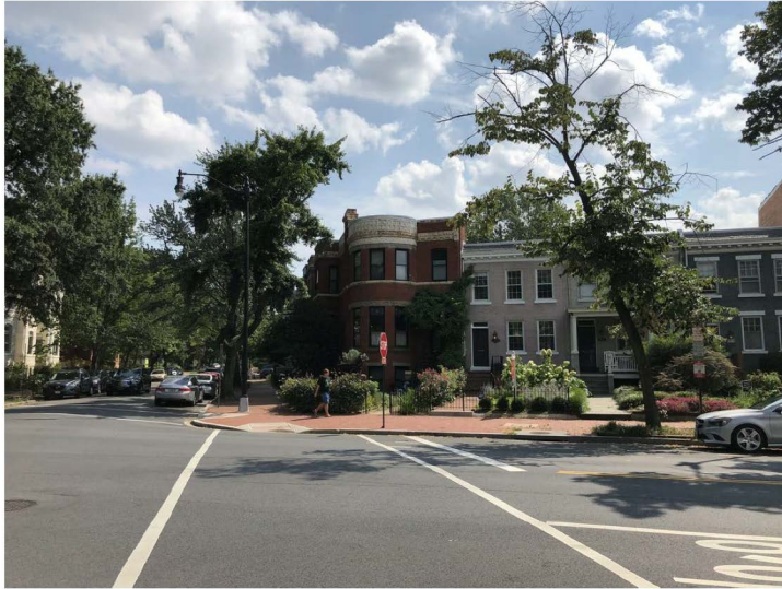
PHOTO A NO ROOFTOP ELEMENTS ARE VISIBLE.
